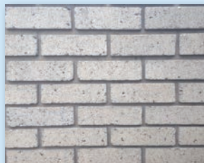
CEMENT STOCK BRICK
