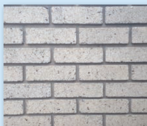
CEMENT STOCK BRICK
