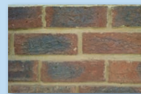
CLAY PLASTER BRICK
