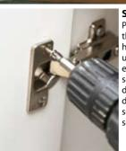
STEP 3 Position the new hinge and use the electric screwdriver to drive the screws in securely.
