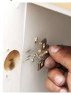
STEP 2 Remove all parts of the old hinge from the door.
